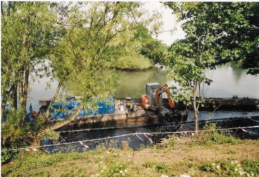
Fig. 4 Placing of “silt” shelf using machinery on floating craft
