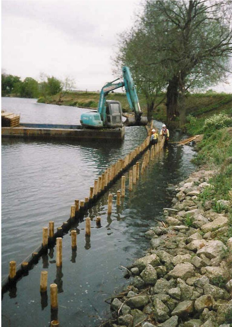
Fig. 5 View of revetment system being placed
