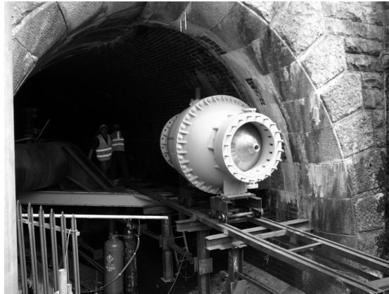
Fig 14: Refurbished valve returning into tunnel.
