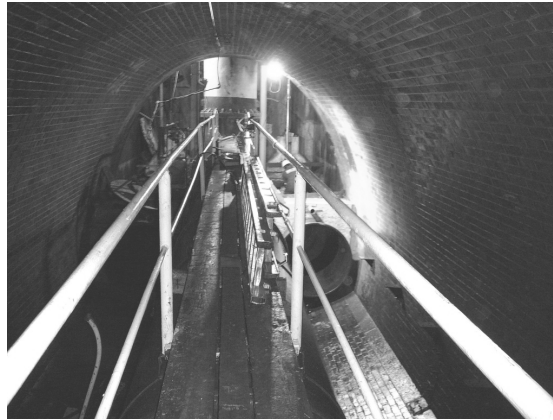
Fig 4: View of bottom of valve tower
