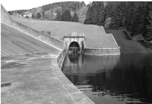
Fig 2: View of tunnel exit and stilling pool
