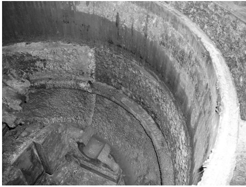
Fig 10: Plunger cavity as found.
