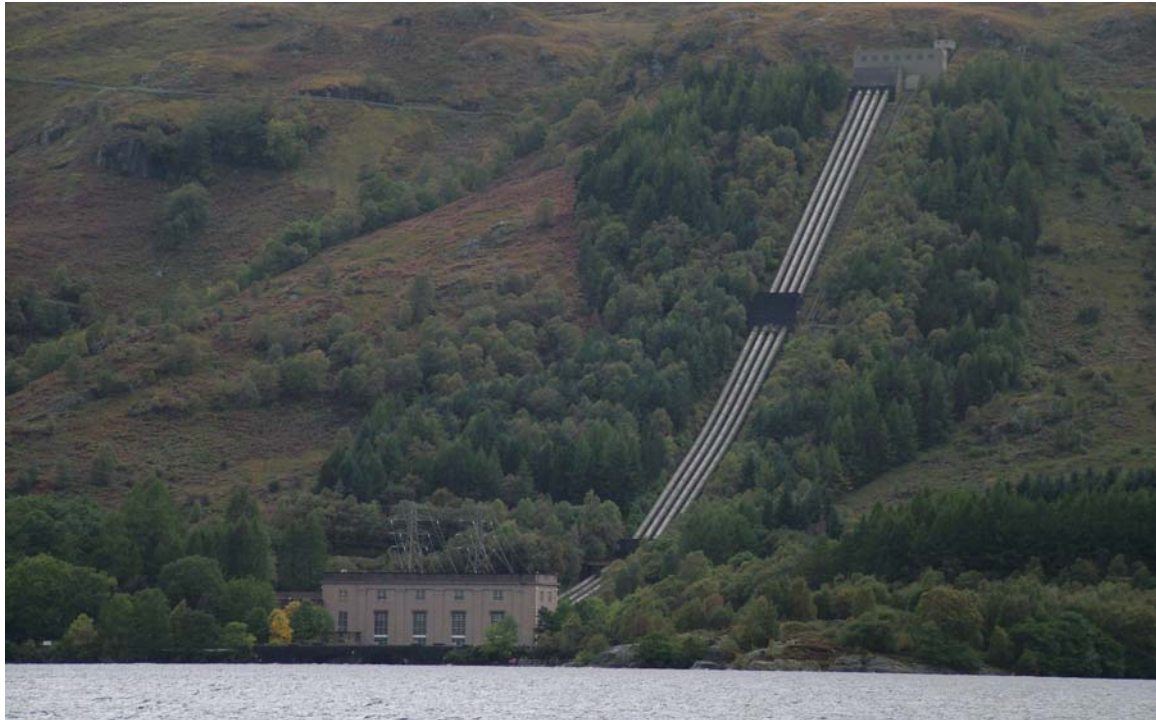
Sloy Power Station
