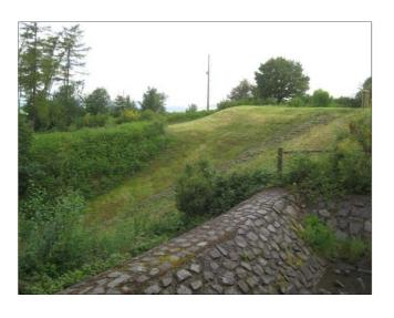
Wet Sleddale, located close to Shap was completed in 1967 to support Haweswater reservoir in supplying water to the Manchester area. The dam is 610m in length and 21m high and retains around 2300m³ of water. The water from the reservoir is transferred via aqueduct, largely constructed as a cut and cover tunnel, to Haweswater itself. The dam is constructed on rock comprising Tuff which was curtain grouted prior to construction of the dam.
